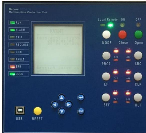
Figure 3.2 The controller (Recloser) device front panel
