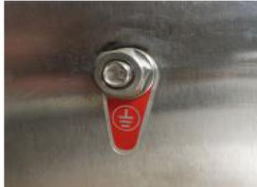
Figure 1-2 The position of the grounding bolt
