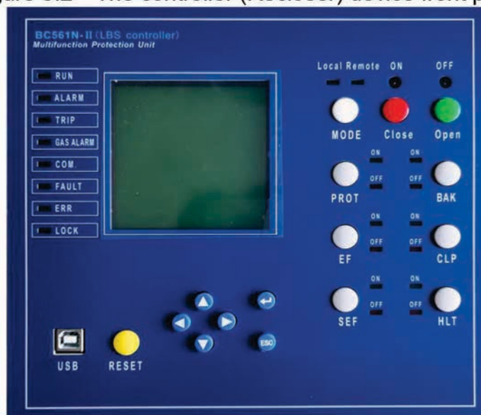
Figure 3.2 The controller (Recloser) device front panel
